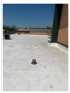
4" metal edge with 22 gauge continuous cleat and covered with Versico cover tape.
